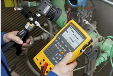
Pressure transmitter calibration
