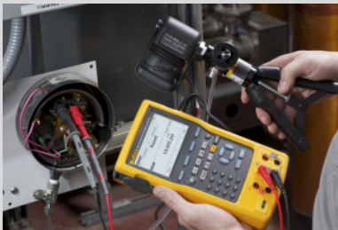
Pressure switch testing
